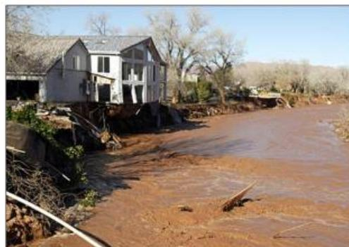
Figure 6. Photos from a 2005 in Saint George Utah, where homes several feet above the mapped floodplain were destroyed by channel migration ([www.Utahfloodrelief.com](http://www.Utahfloodrelief.com)).
