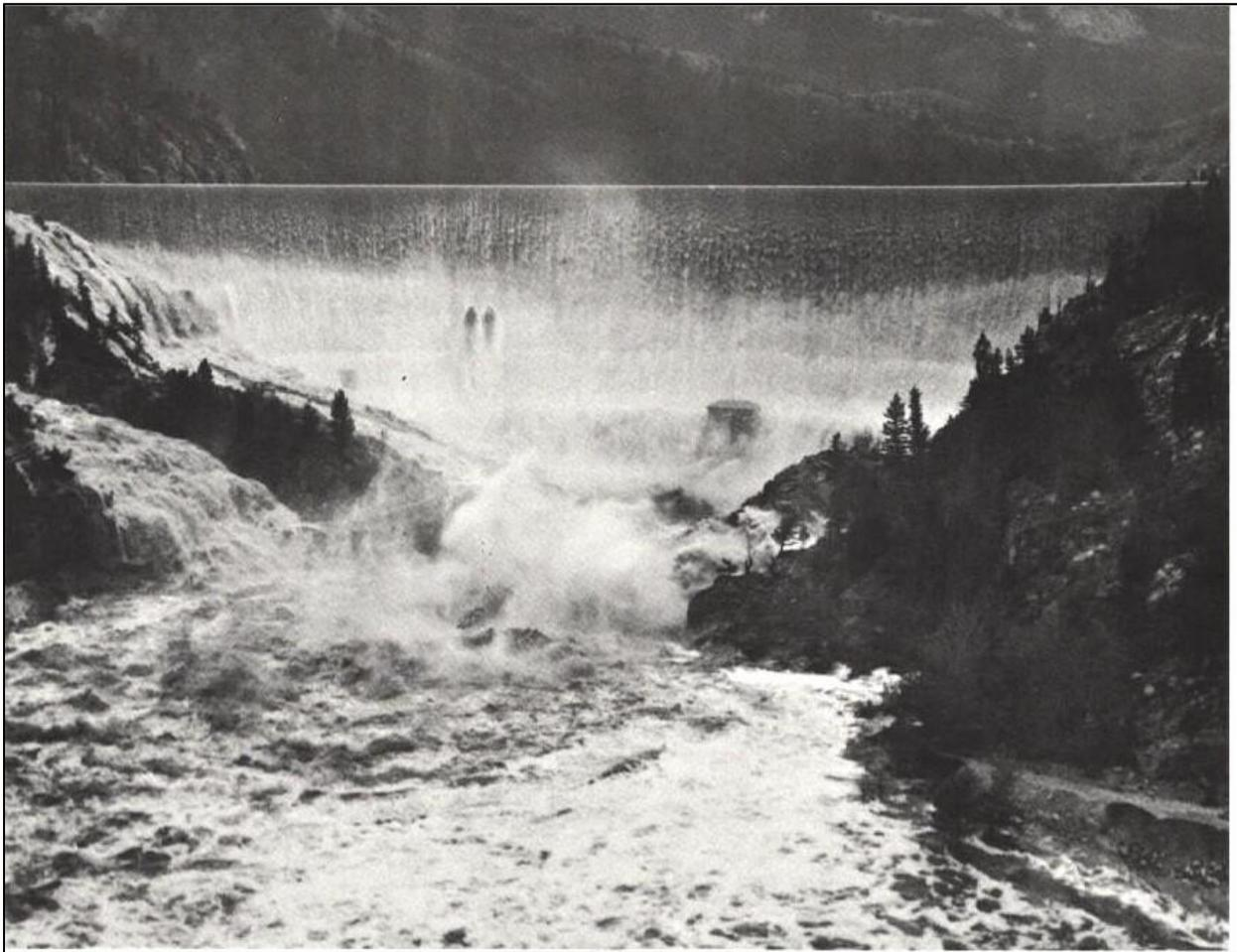
**Figure 25. Gibson Dam overtopping with over 3 feet of water on the dam crest during 1964 flood (USGS).**
