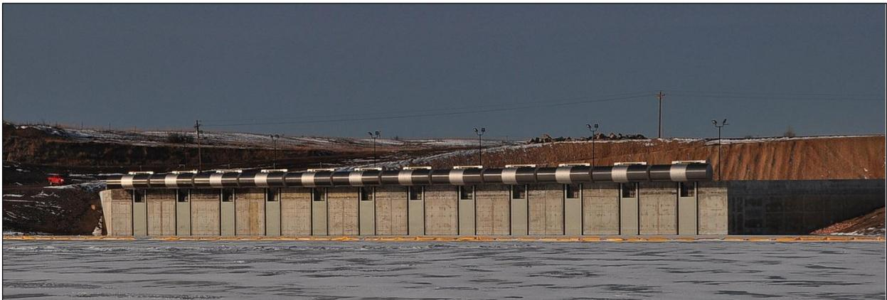
Figure 4-31 New headworks with fish screens, Intake Diversion (USBOR)
