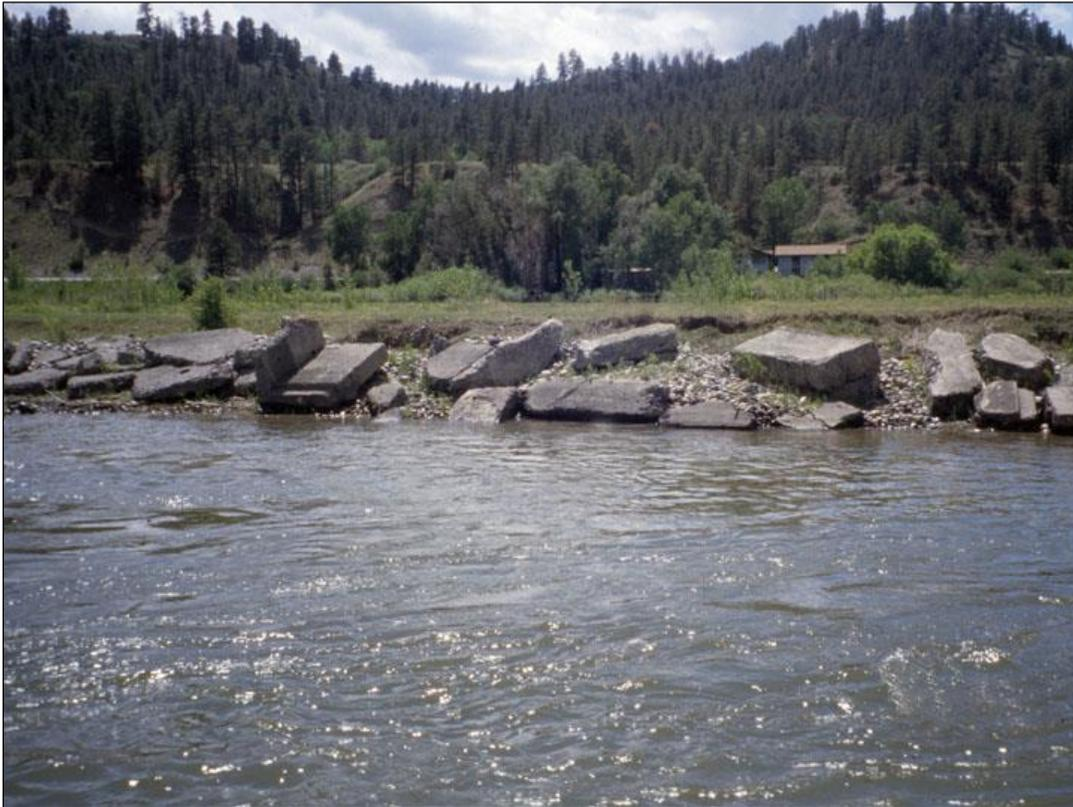
**Figure 8-4** Concrete blocks dumped on the riverbank are ineffective and will likely accelerate the rate of bank erosion, rather than prevent it
