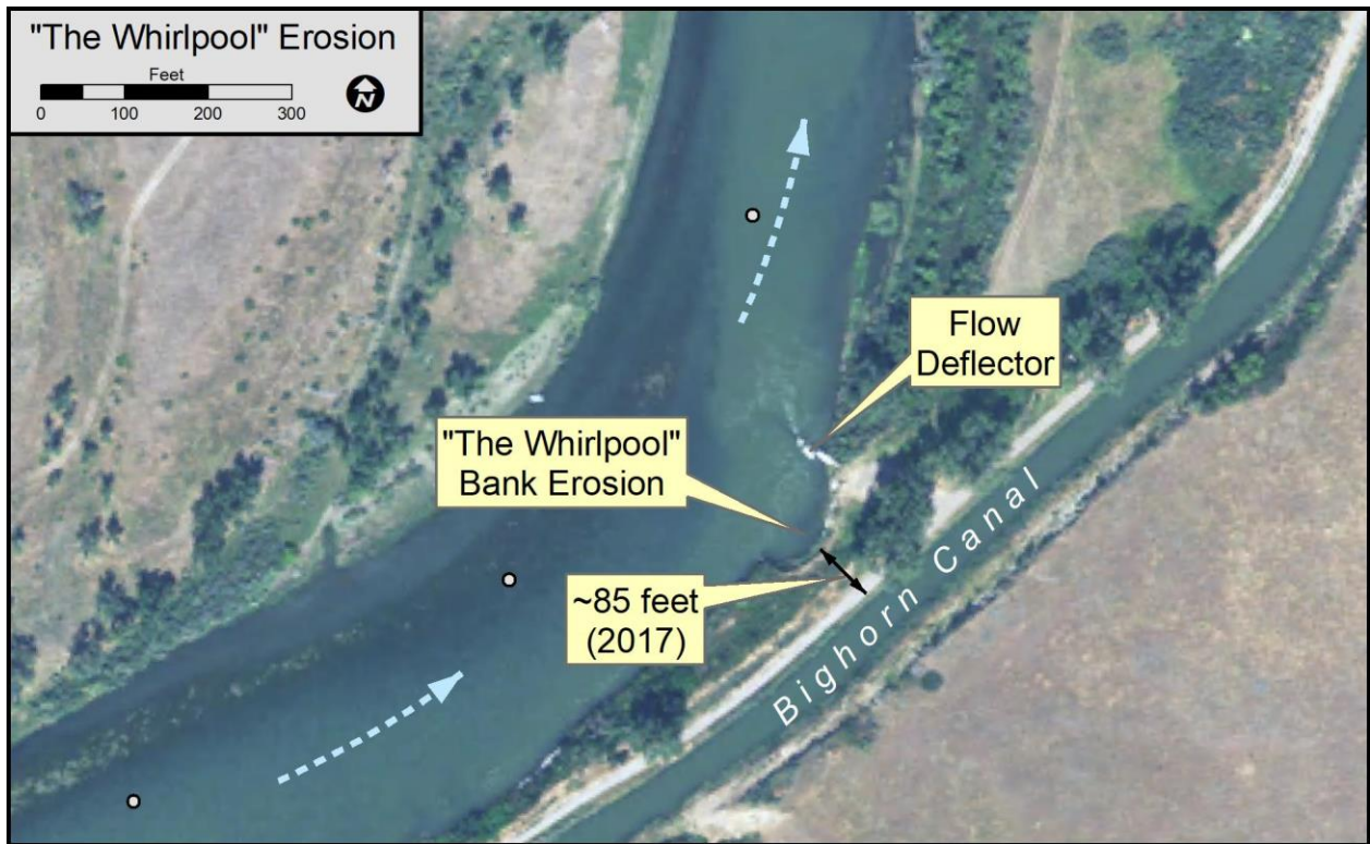
Figure 43. 2017 air photo showing scour upstream of flow deflector; back eddy has eroded the bank towards Bighorn Canal.
