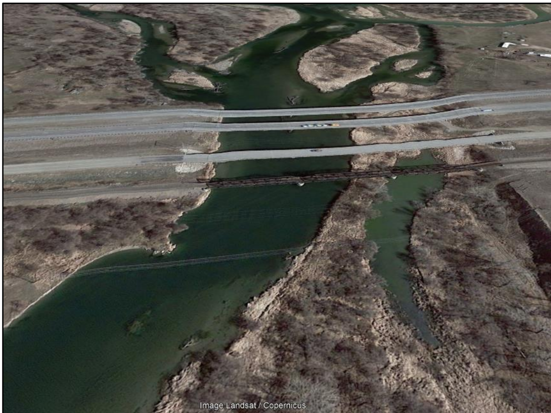
Figure 63. Google Earth image showing flanking of left bank armor above Interstate Bridge.
