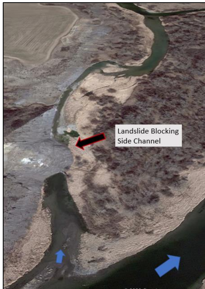
Figure 9. Google Earth (2016) image showing side channel blocked by landslide at RM 56.7.
