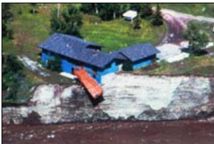
Figure 5. Yellowstone River home on high glacial terrace that was burned down in 1997 to prevent its undermining by the river.
