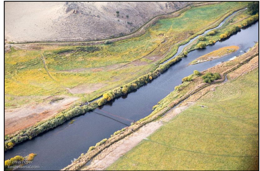
Figure 76. Local access bridge (RM 16.9), September 30, 2017 (Kestrel).
