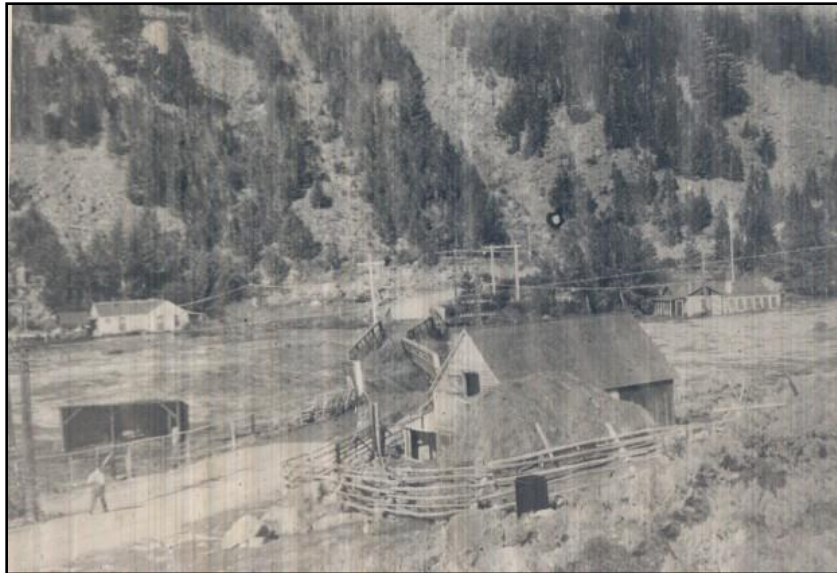
Figure 13. 1927 photo of Big Hole River Bridge washout following Pattengail Reservoir failure.
