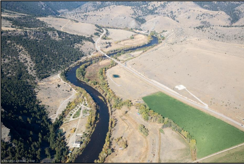
Figure 85. Hwy 43 bridge at Divide, October 6, 2017 (Kestrel).
