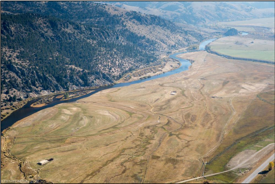
Figure 46. View downstream of Reach BH9 showing overflow paths on 100-year floodplain, RM 65.0. (Kestrel)
