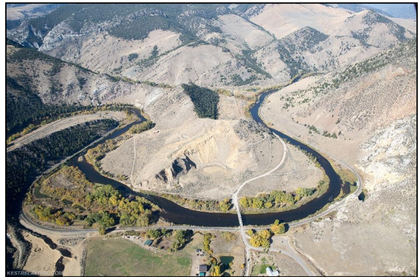
Figure 84. Maiden Rock Road bridge, October 6, 2017 (Kestrel).
