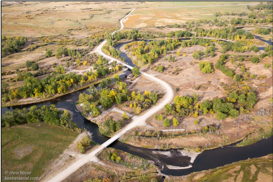
Figure 61. View west showing two Burma Road Bridges; far bridge approach angle has decayed with time and road is increasingly threatened. (Kestrel)
