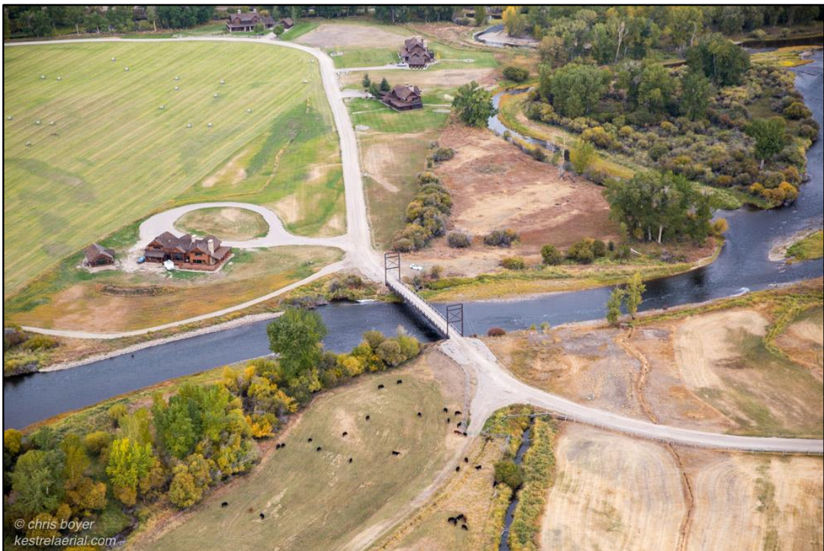
Figure 54. Meriwether Ranch housing development on Big Hole River island, Reach BH5. (Kestrel)
