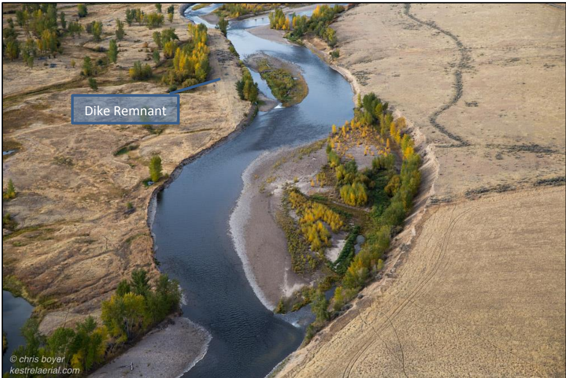
Figure 72. View upstream of high left bank terrace above High Bridge; note breached dike remnant on right bank.
