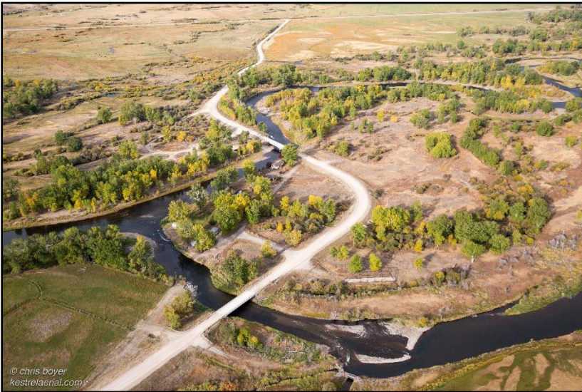
Figure 78. Burma Road bridges, September 30, 2017 (Kestrel).
