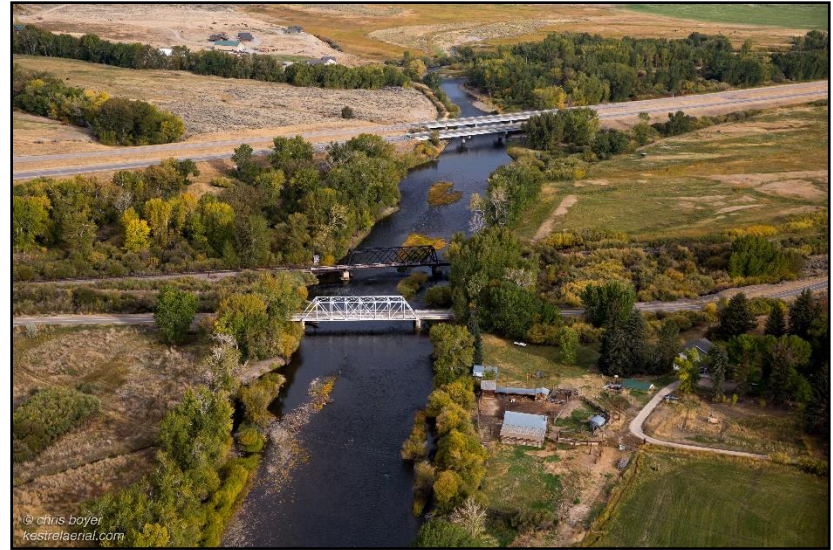
Figure 79. Hwy 91, railroad, and I-15 bridges, September 30, 2017 (Kestrel).
