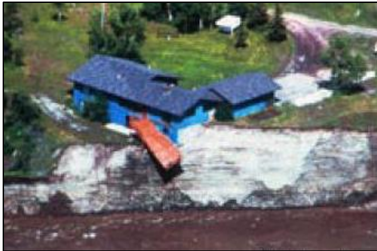
Figure 4. Yellowstone River home on high glacial terrace that was burned down in 1997 to prevent its undermining by the river.
