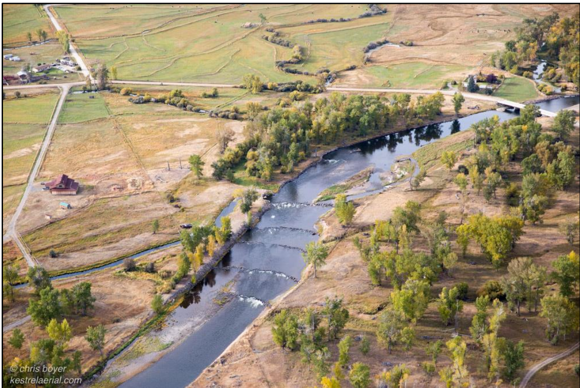
Figure 71. View upstream of rock grade controls at diversion structure just below Pennington Bridge.
