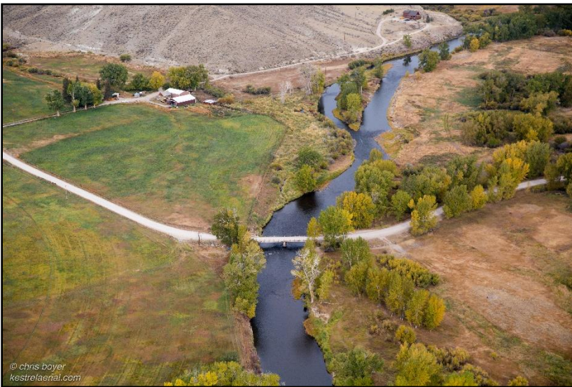
Figure 82. Trapper Creek Road west bridge, September 30, 2017 (Kestrel).
