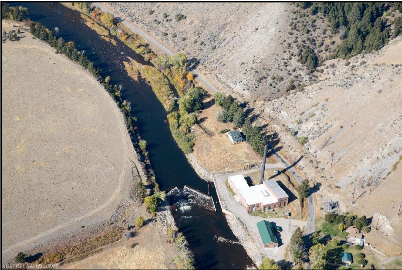
Figure 86. Pump house diversion, October 6, 2017 (Kestrel).
