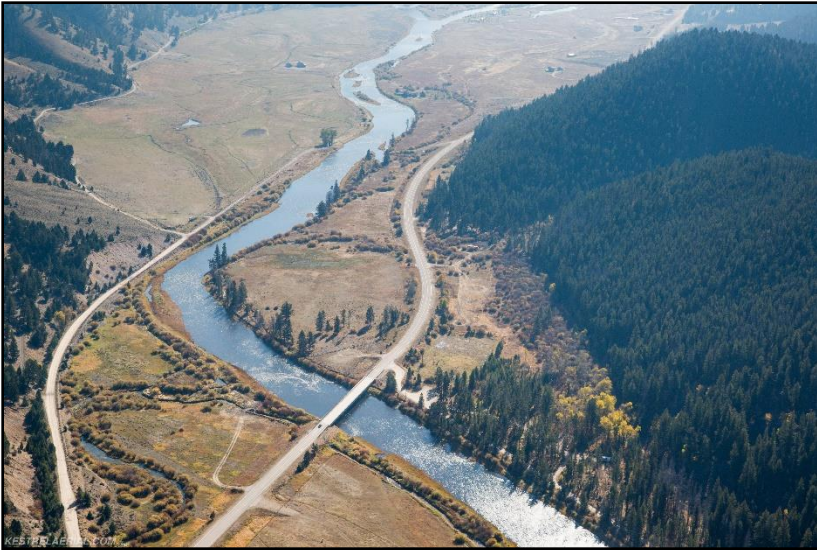
Figure 89. Dickie bridge, October 6, 2017 (Kestrel).
