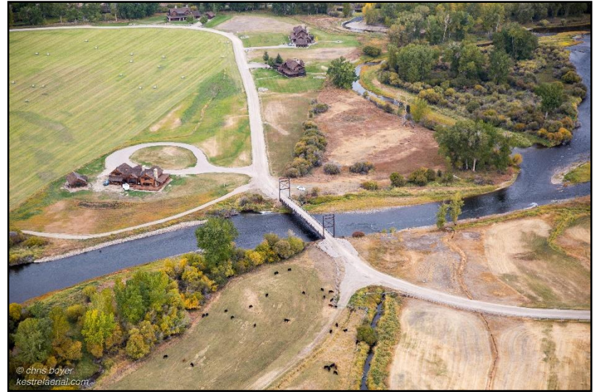
Figure 83. Meriwether Ranch bridge, September 30, 2017 (Kestrel).
