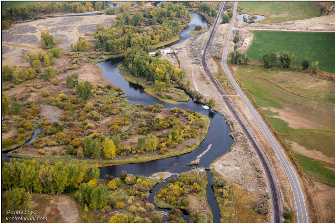
Figure 53. View upstream showing channel migration towards the railroad grade near Melrose, RM 37.3.
