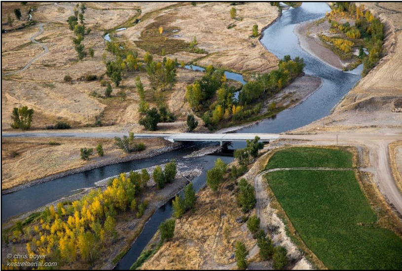
Figure 73. High Bridge, September 30, 2017 (Kestrel).
