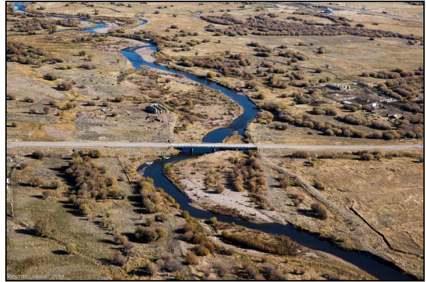
Figure 91. Hwy 43 bridge at Wisdom, October 6, 2017 (Kestrel).
