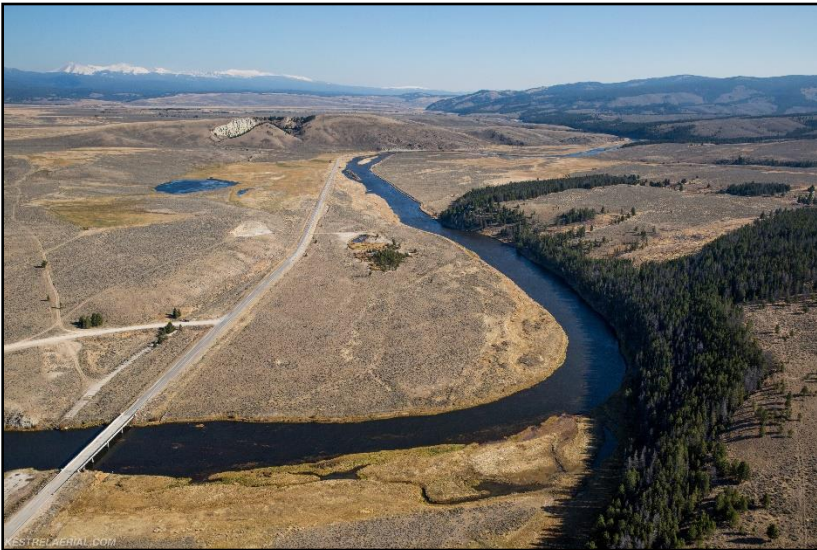
Figure 90. Hwy 43 bridge at N Fork Road, October 6, 2017 (Kestrel).
