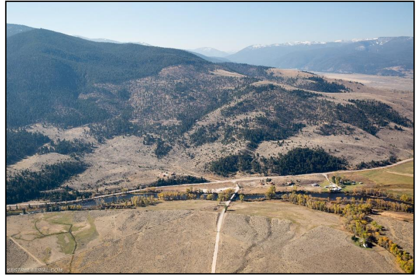
Figure 87. Jerry Creek Road bridge, October 6, 2017 (Kestrel).
