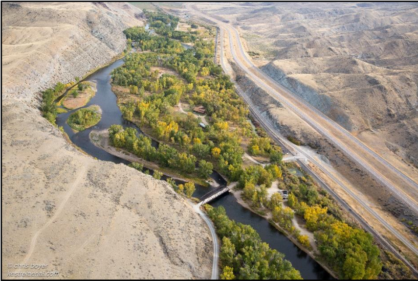
Figure 81. Browns Bridge Road, September 30, 2017 (Kestrel).
