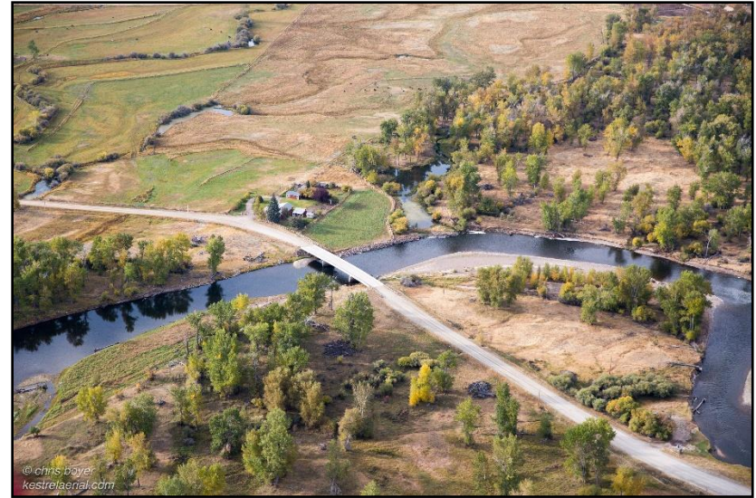
Figure 75. Pennington Bridge, September 30, 2017 (Kestrel).
