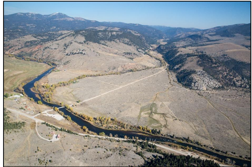
Figure 88. Jerry Creek Road bridge, October 6, 2017 (Kestrel).
